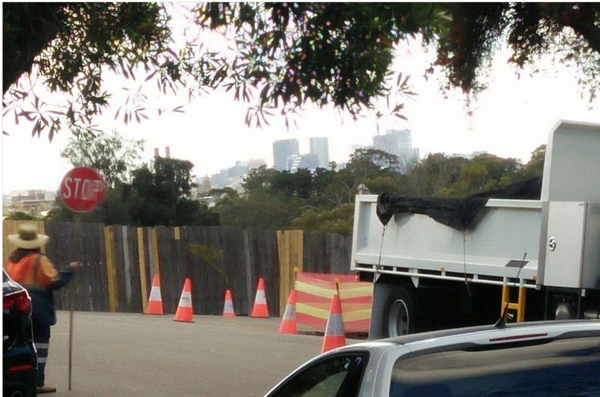
Figure R – View from front yard of No. 32 Emma Street (photo from objector)
