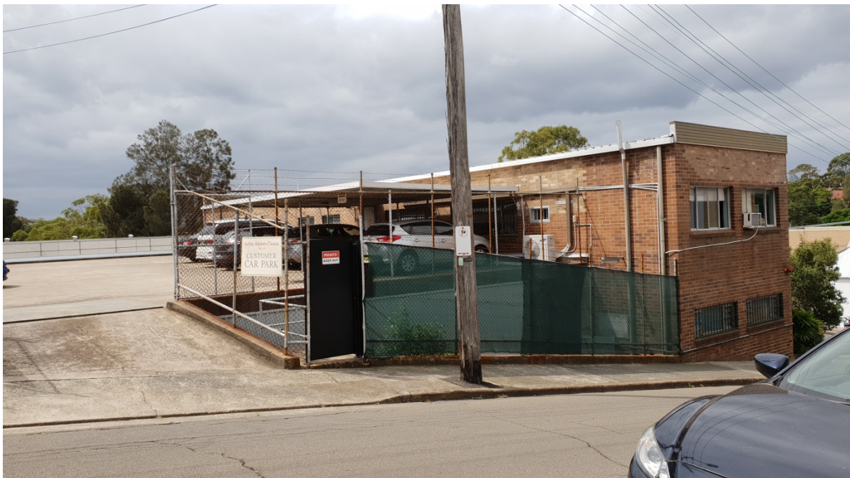
View of existing building from Hill Street.
