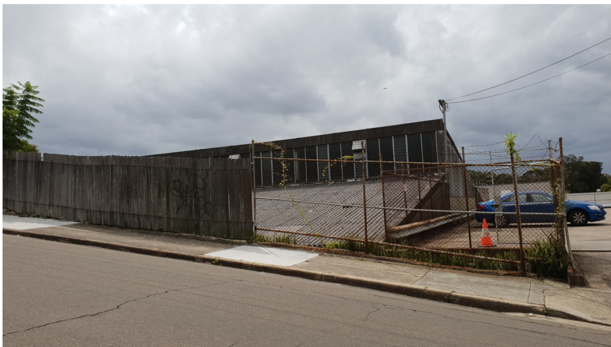
View of existing building from Hill Street.
